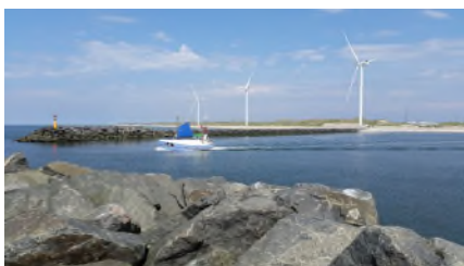
Figure 36: Wind turbines in Hvide Sande owned by local citizens/companies, supplying the heat pump in the district heating with green electricity.
