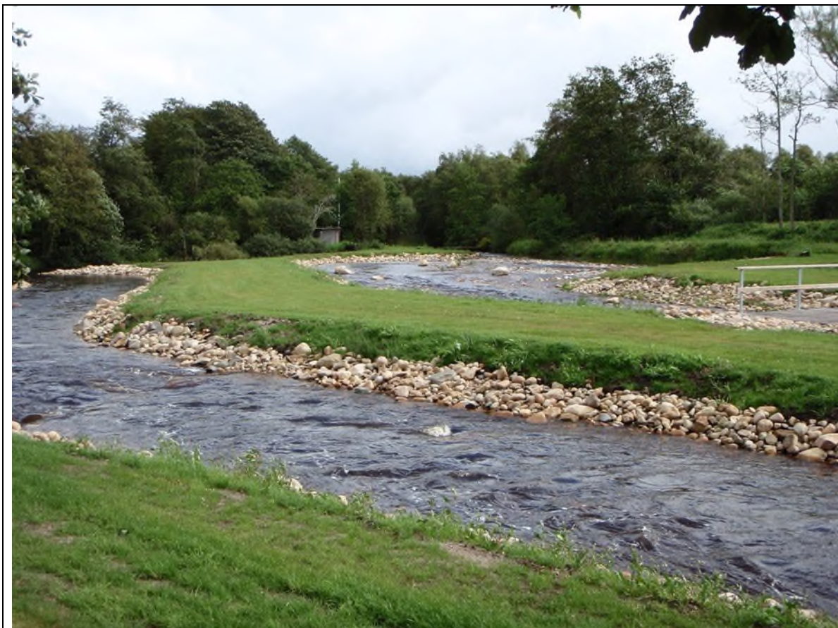
Figure 33: Successful watercourse restoration. Bypass flow by Hoven Watermill.
