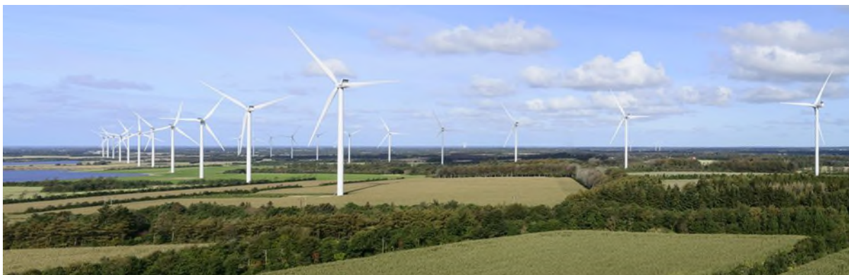
Figure 4: Nørhede-Hjortmose is Denmark's largest on-shore energy park with 22 wind turbines 150m in height and 26ha photovoltaics
